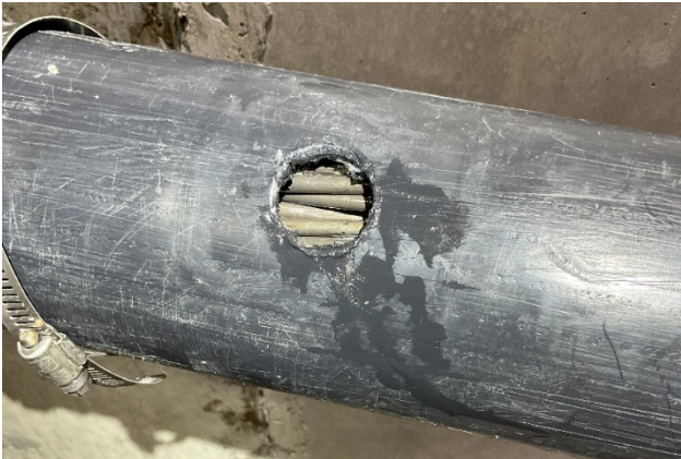
Figure 18: Side of Tendon Opened and Prepared for Port Installation
