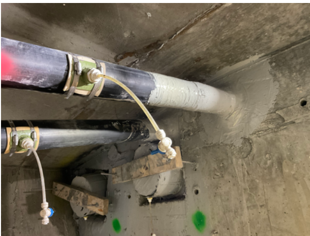
Figure 19: Tendons and Anchor Caps Ported.
