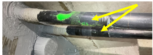
Figure 22: Repaired Port Locations After PTI Impregnation
