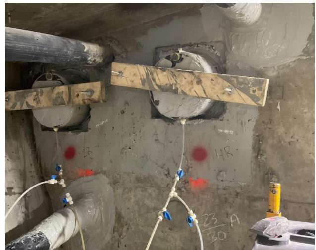
Figure 17: Grout Cap Installed with Impregnation Port
