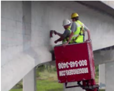
Figure 1: Locating PT tendons using GPR
