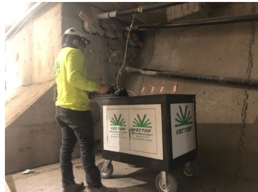
Figure 21: PTI Technician Monitoring the Impregnation of a Tendon
