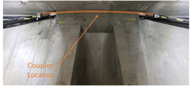
Figure 15: Tendon across diaphragm - Condition 1
