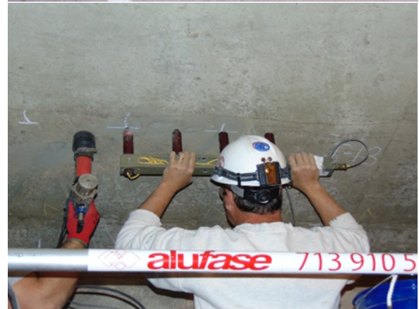
Figure 5: Sonic/Ultrasonic Testing of PT Tendons
