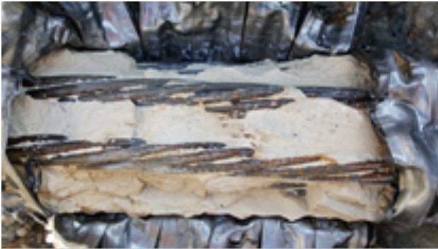
Figure 6: PT Tendon Opening
