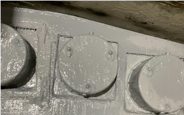
Figure 23: Repaired Grout Caps Sealed with Elastomeric Coating after PTI Impregnation
