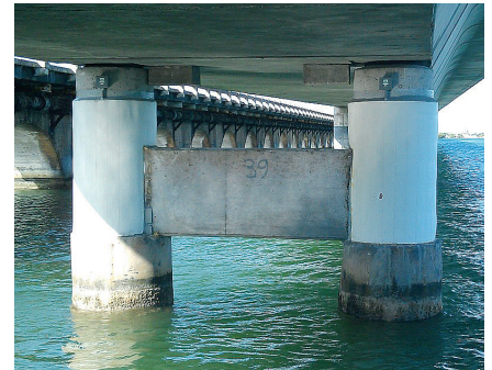
Galvashield DAS Jackets provide protection to pile sections above the tidal zone.
