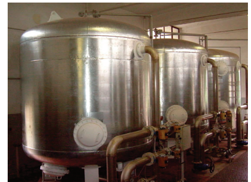
Condition of Tanks after ZincTape Application
