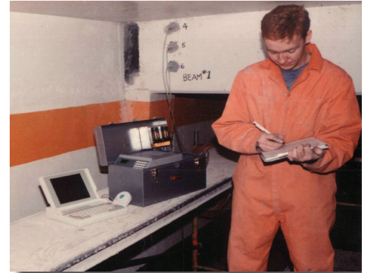
Post-Tech PT Corrosion Evaluation of Cables
