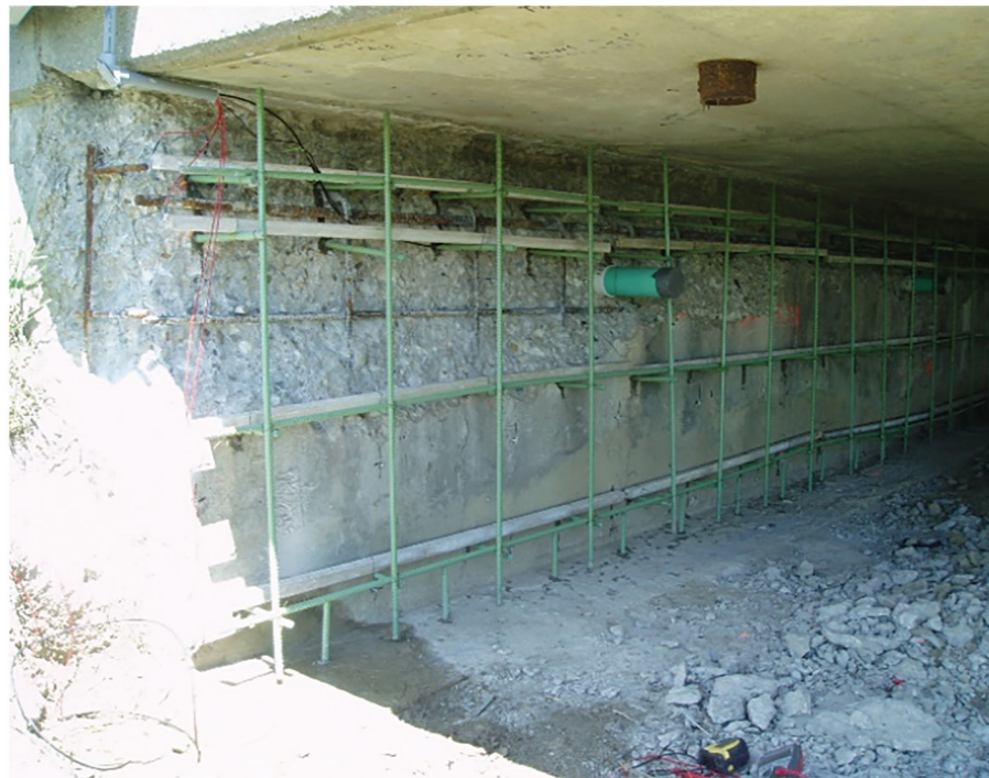
FIGURE 1 Galvanic encasement of abutment using distributed galvanic anodes, Sidney, Ohio.
