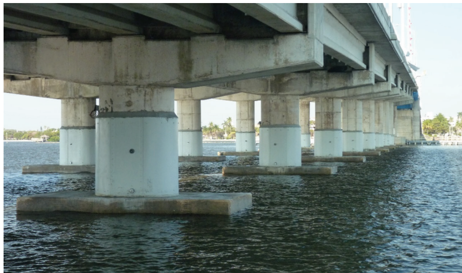
FIGURE 2 New distributed anode cathodic protection jackets installed, Lake Worth, Florida.
